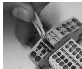
Remove shunt to deactivate a heater (reduction of 1000 W)
